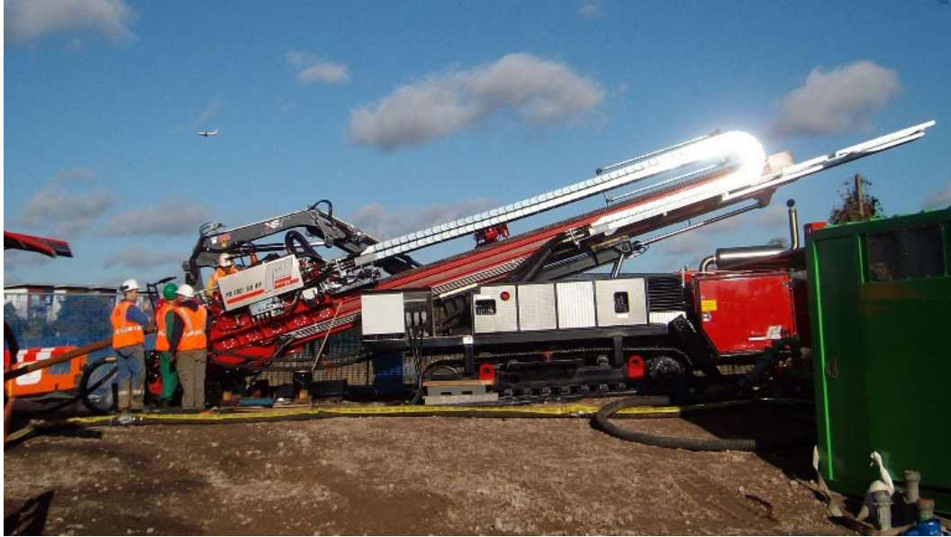
Figure 4.7: Photo of Typical maxi-rig HDD Drill Rig
