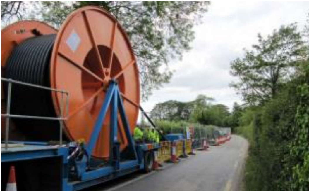
Figure 4.13: Cable Drum at Joint-bay location
